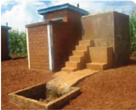
Picture 7: Pit latrine with rain harvest tank / hand washing facility, Tenecha CBCC
